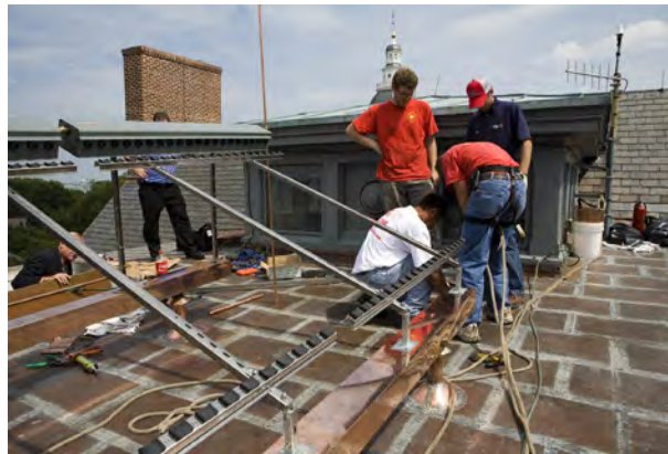
Workers install solar panel atop Government House as part of the DGS Energy Performance initiatives at 37 DGS-operated buildings.
