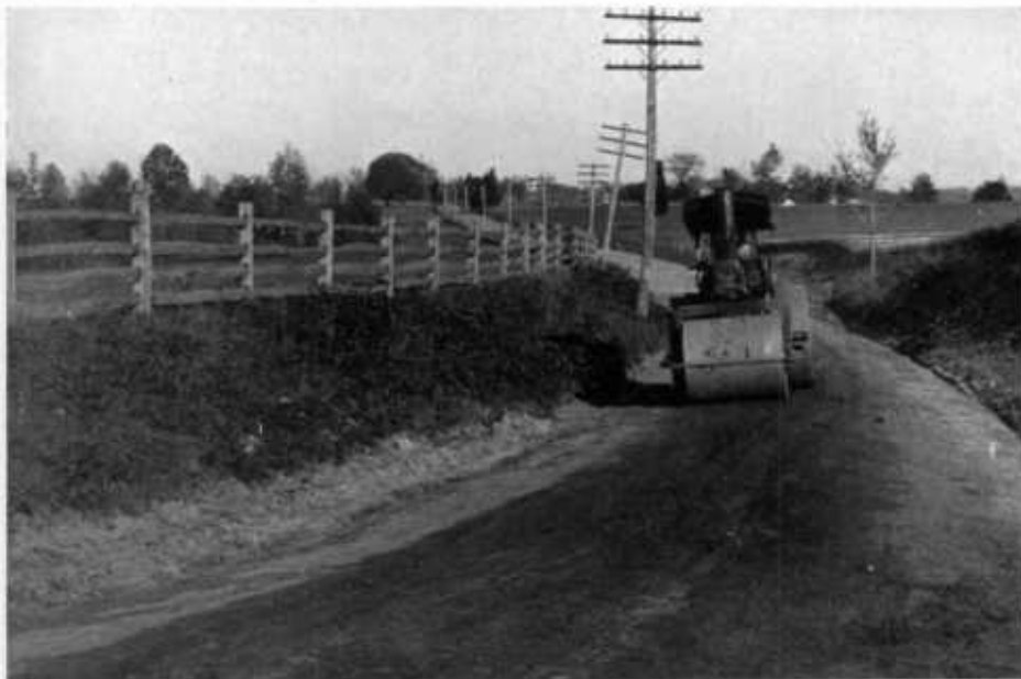
FIG. 1.—BELAIR—CHURCHVILLE ROAD, HARFORD COUNTY. FINISHING A MACADAM ROAD.
