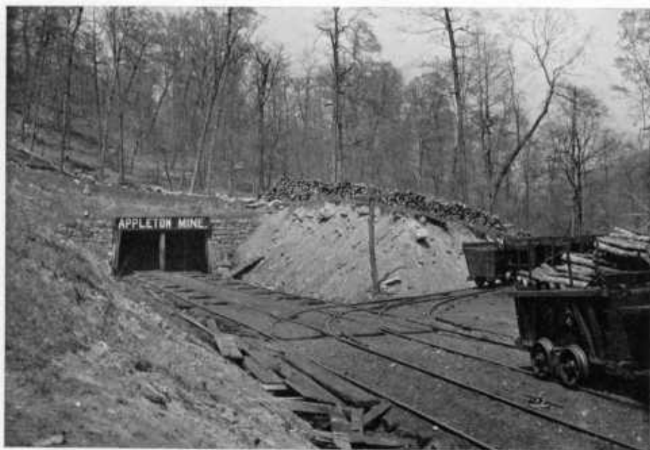
FIG. 2.—MARYLAND COAL COMPANY, APPLETON.
