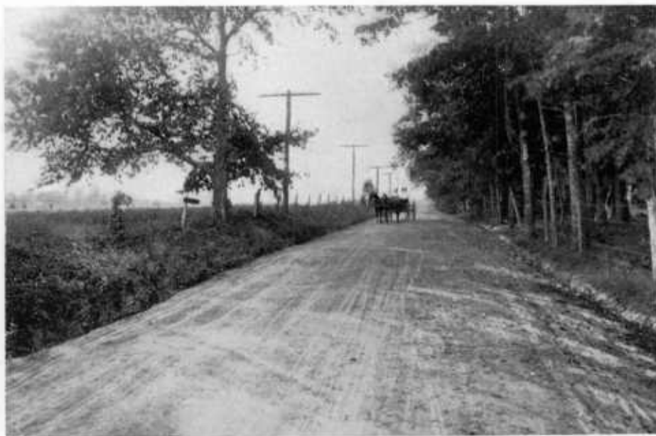
FIG. 2.—CHESTERTOWN—CENTERVILLE ROAD, QUEEN ANNE'S COUNTY. SLAG ROAD NEAR CHESTERTOWN.
