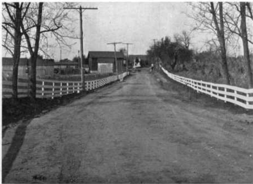
FIG. 2.—RISING SUN-FARMINGTON ROAD, CECIL COUNTY. MACADAM ROAD, ALL COURSES MADE OF TRAP ROCK.
