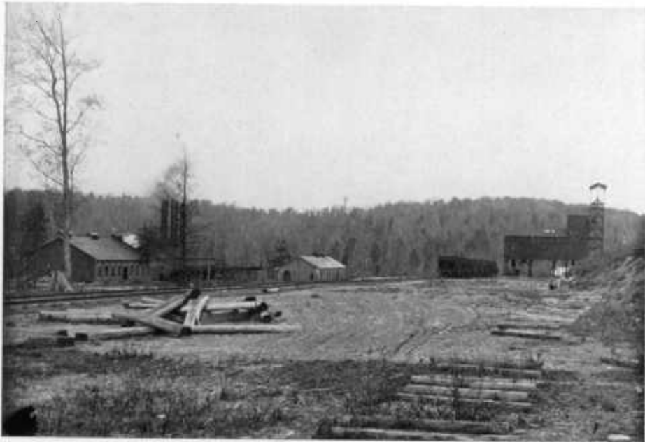
FIG. 2.—DAVIS COAL AND COKE COMPANY, HENRY.
