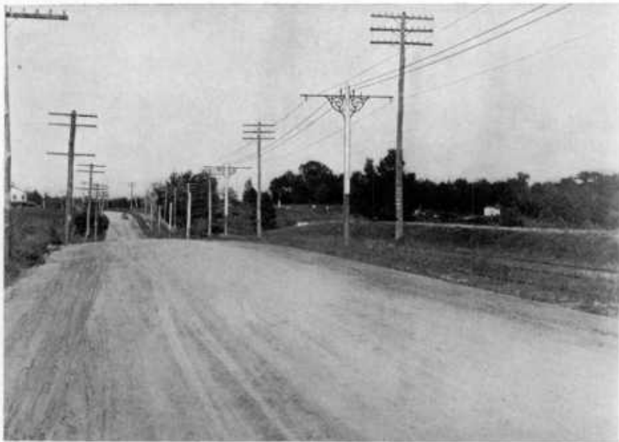
FIG. 1.—EASTERN AVENUE, BALTIMORE COUNTY. MACADAM ROAD WITH TRAP ROCK TOP AND SLAG FOUNDATION, SLAG SCREENINGS USED FOR "BINDER".
