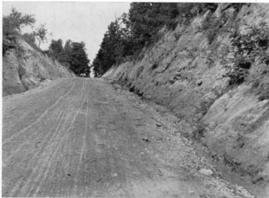
FIG. 1.—T B ROAD, PRINCE GEORGE'S COUNTY. DEEP CUT MADE TO REDUCE THE GRADE OF WILSON'S HILL.
