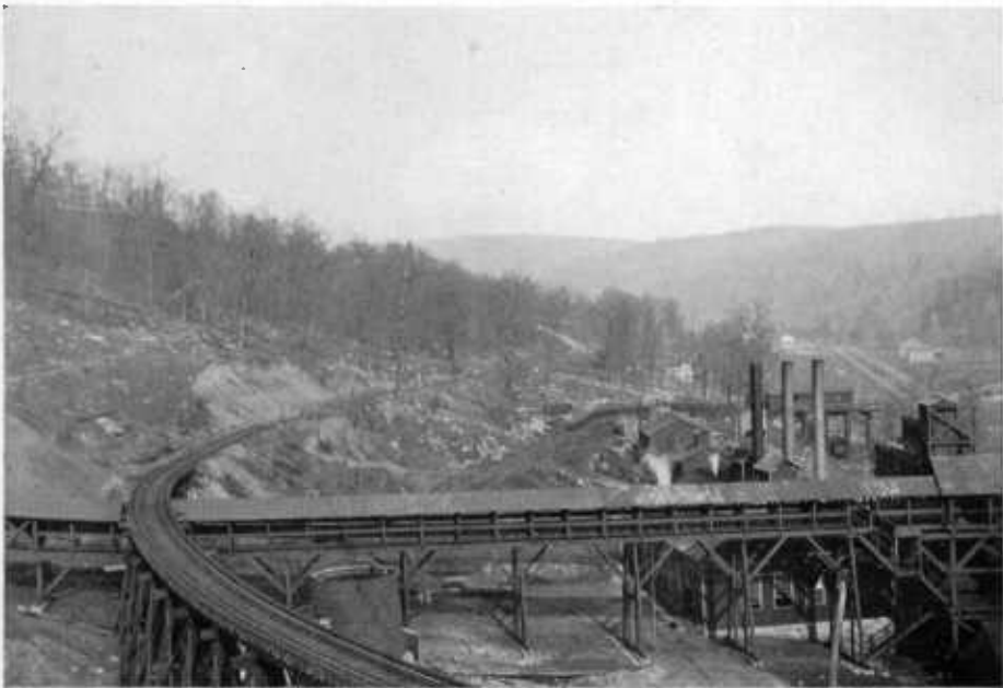
FIG. 2.—GEORGES CREEK COAL AND IRON COMPANY, GILMOR.
