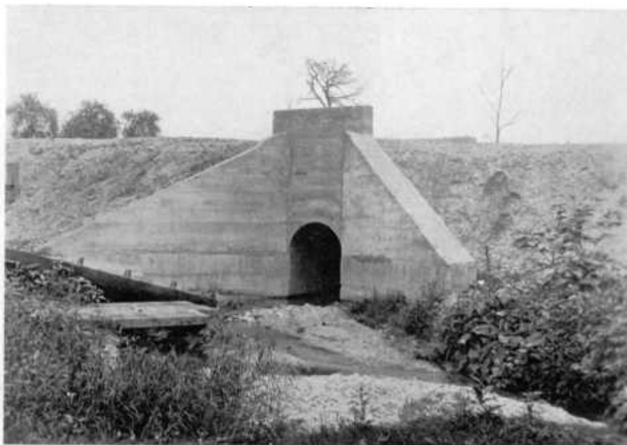
FIG. 2.—T B ROAD, PRINCE GEORGE'S COUNTY. CONCRETE CULVERT AND EMBANKMENT AT THE FOOT OF WILSON'S HILL.
