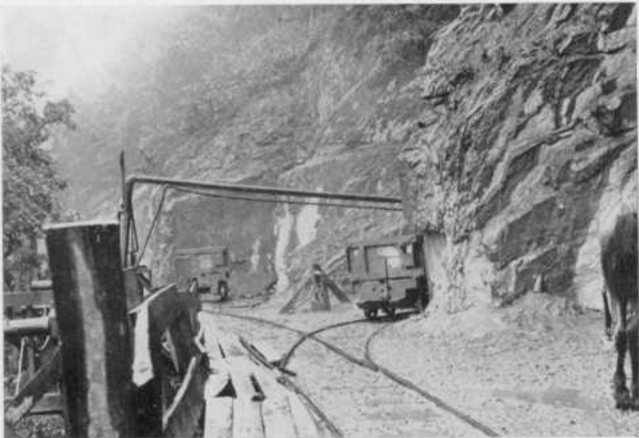
FIG. 2.—QUARRY OF CUMBERLAND AND POTOMAC CEMENT COMPANY, POTOMAC.
