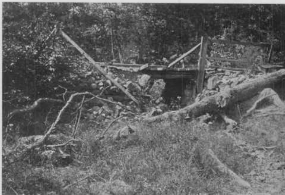
FIG. 1.—OLD CULVERT ON RIVER ROAD BETWEEN CUMBERLAND AND CRESAPTOWN, ALLEGANY COUNTY.
