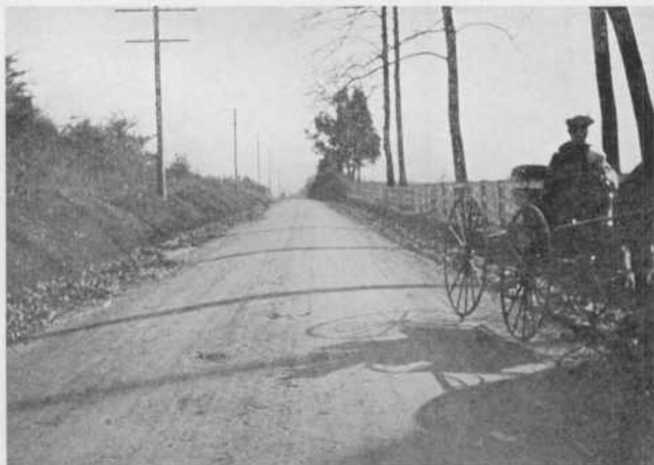
FIG. 2.—CHESAPEAKE AVENUE, BALTIMORE COUNTY, AFTER IMPROVEMENT BY COUNTY ROADS ENGINEER.
