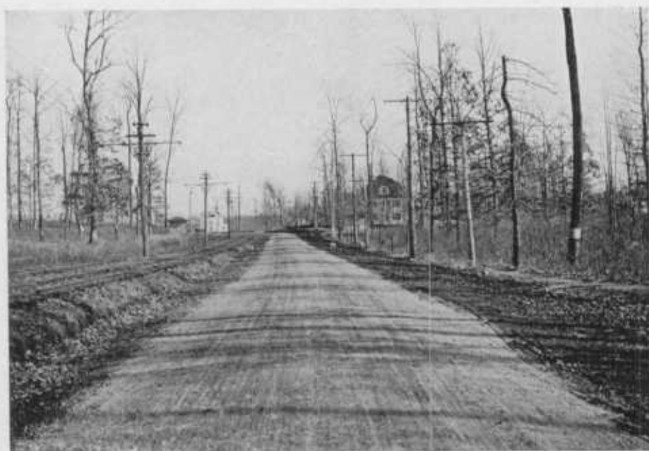
FIG. 2.—SECTION OF GWYNN OAK AVE., BALTIMORE COUNTY, AFTER IMPROVEMENT UNDER STATE AID.
