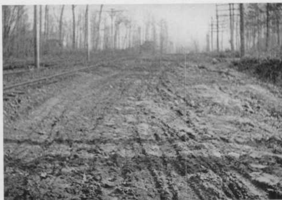
FIG. 1.—SECTION OF GWYNN OAK AVE., BALTIMORE COUNTY, BEFORE IMPROVEMENT.
