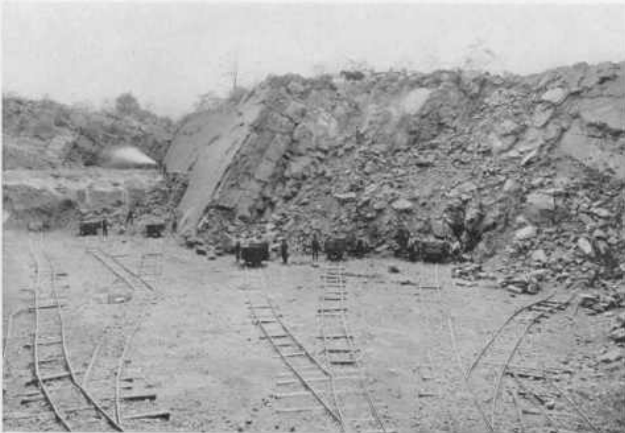
FIG. 2.—QUARRY OF POTOMAC VALLEY STONE AND LIME COMPANY, PINESBURG.
