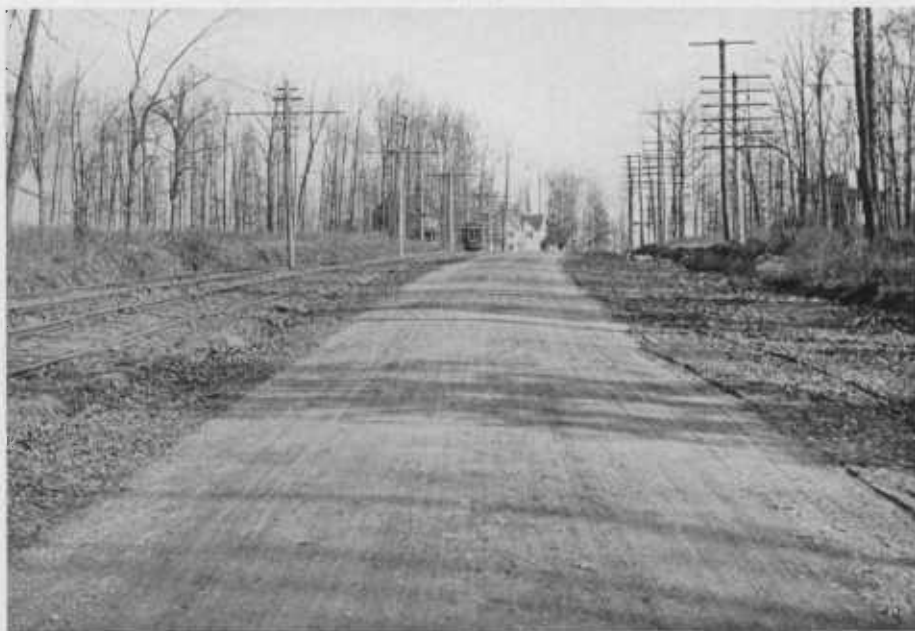
FIG. 2.—SECTION OF GWYNN OAK AVE., BALTIMORE COUNTY, AFTER IMPROVEMENT UNDER STATE AID.
