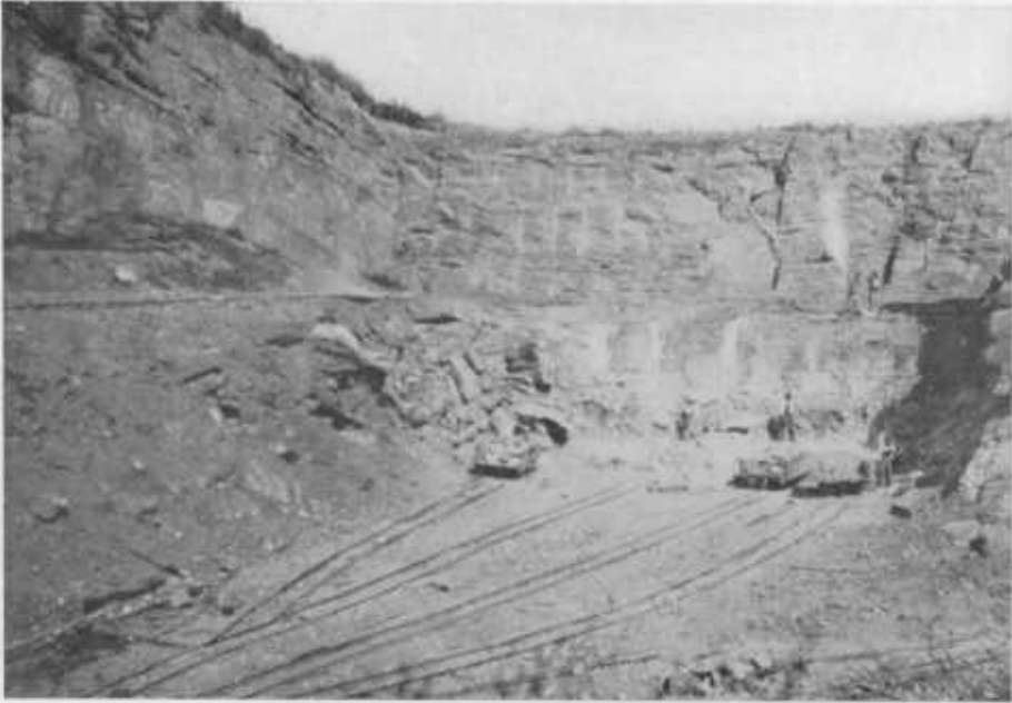
FIG. 1.—QUARRY OF S. P. ANGLE, HAGERSTOWN.
