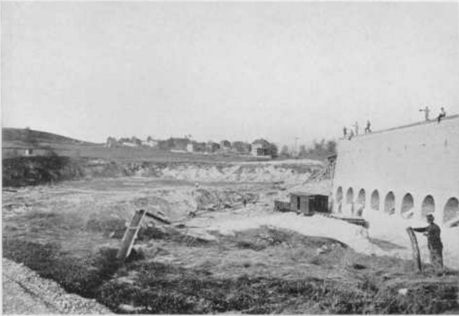
FIG. 1.—KILNS AND QUARRY OF S. W. BARRICK & SONS, LE GORE.
