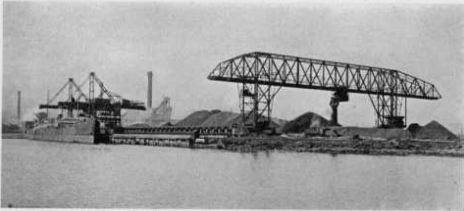
FIG. 64.—ORE DOCKS AT SPARROWS POINT.
