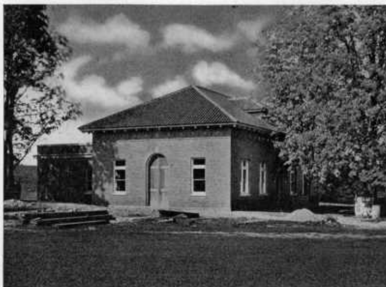
FIG. 95.—VIEW OF UPPER SERVICE PUMPING STATION.
