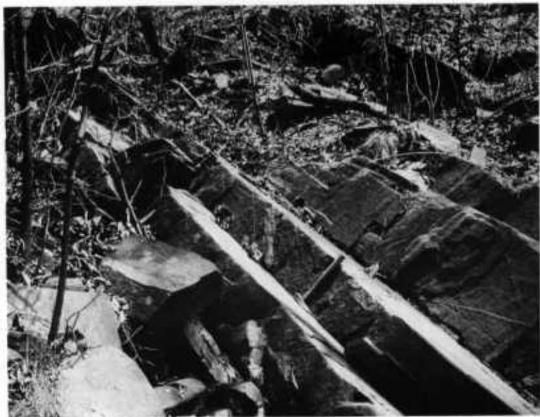
FIG. 2.—Cross jointing. Patapsco River, one mile southeast of Hollofield.
