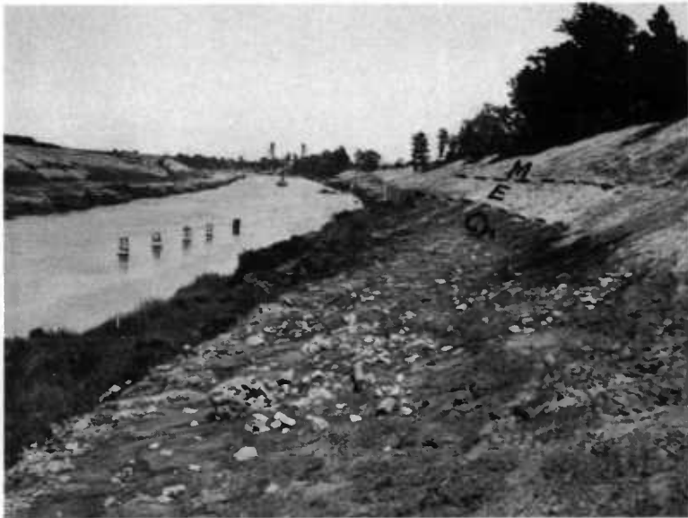
FIG. 2.—The canal east of Summit Bridge, Delaware, during the recent dredging operations. M = Marshalltown; E = Englishtown; Cr = Crosswicks.
