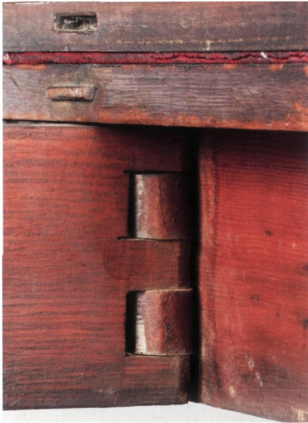
Figure 24 Detail of the fly rail hinge and alignment mortise and tenon on the leaves of the card table illustrated in fig. 21. (Photo, Gavin Ashworth.)
